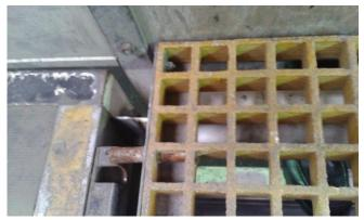
We recently experienced an incident where an operative fell into a cone well whilst loading a stationary IPV, resulting in bruising and minor ligament damage. When the operative accessed the vehicle he believed that the well cover was in place and correctly secured. On investigation it appears that the well cover supports were not correctly located in their retaining slots. The cone well cover was therefore not correctly secured & subsequently dropped into the cone well.
